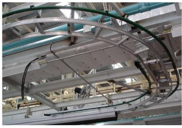
Exhaust Extraction System on a Final Assembly Line
