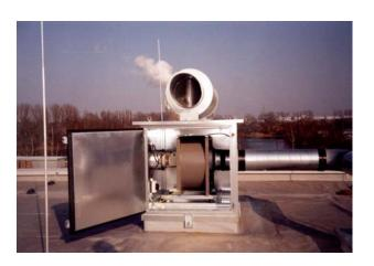
Fans installed in Wether Proof Sound Damping Box on the Roof
